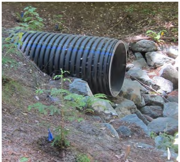
Left: Poles protect a culvert inlet from branches and sediment; Right: Culvert with rocks at outlet for energy dissipation
